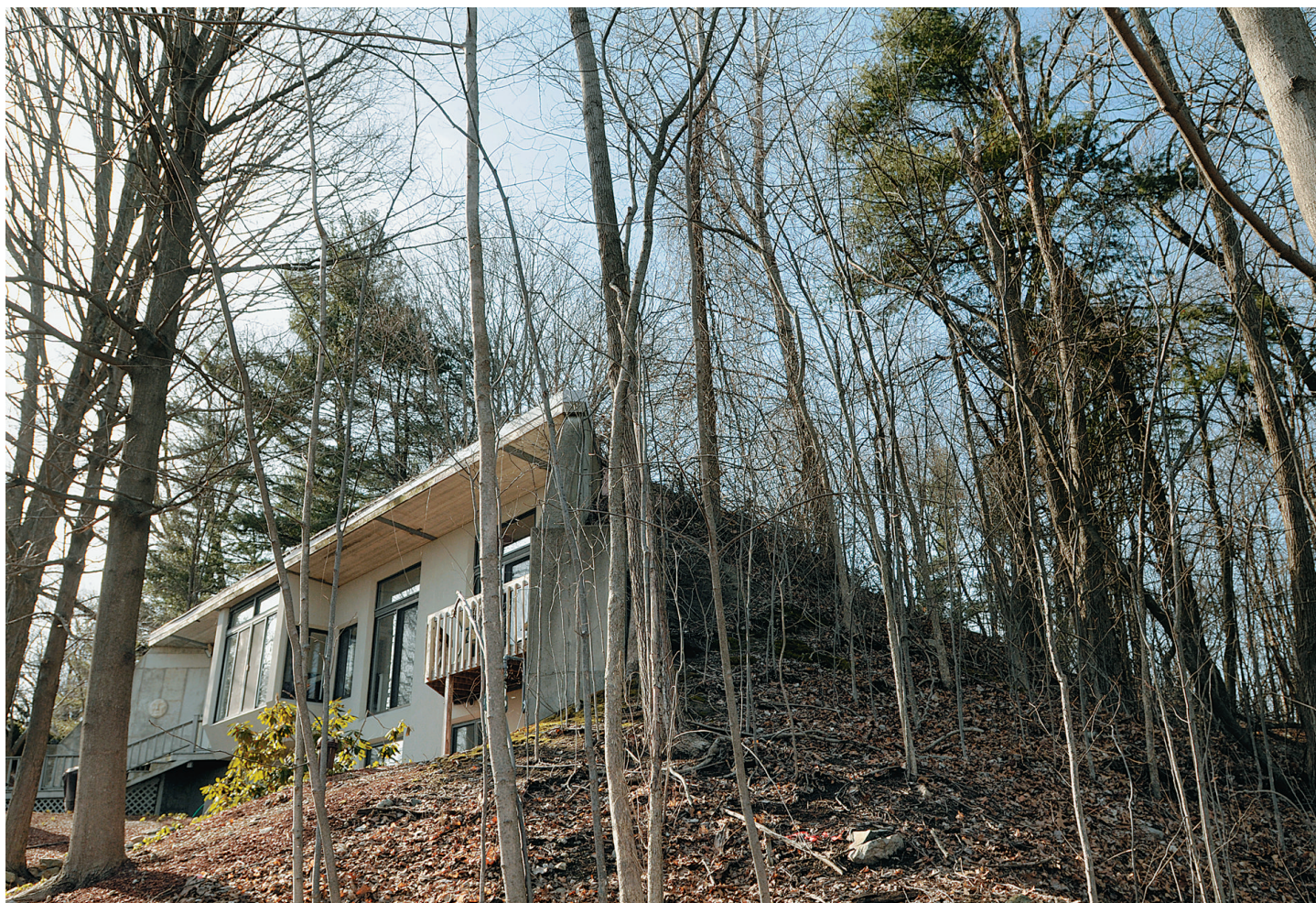
Three walls of the Leinbach-Linton home are built into the hillside. The one exterior wall blends into the landscape.
