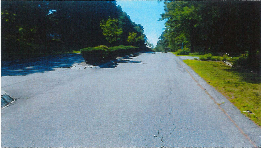
Picture-2. View from opening at 4 Davis Rd toward Ashley Rd
