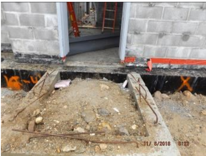
Photo depicts the completion of footings at entry doors, and door frames at CMU walls.
