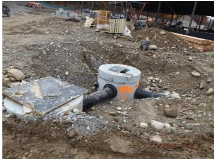
Photo depicts the installation of site drainage.
