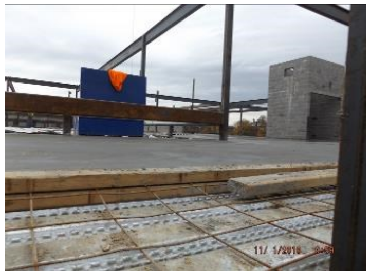
Photo depicts the cured second floor concrete deck.
