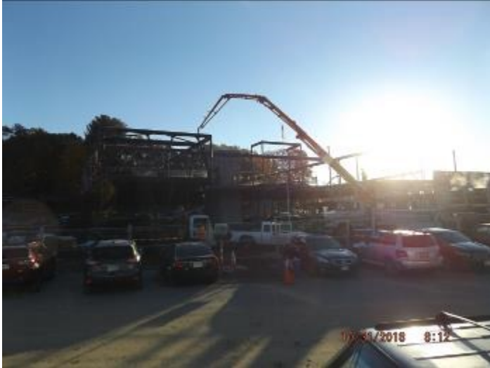
Photo depicts the second floor concrete deck being poured
