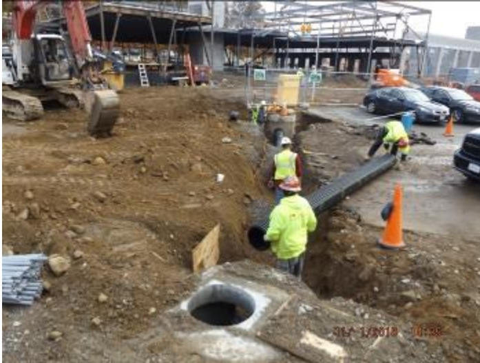
Photo depicts the installation of site drainage.
