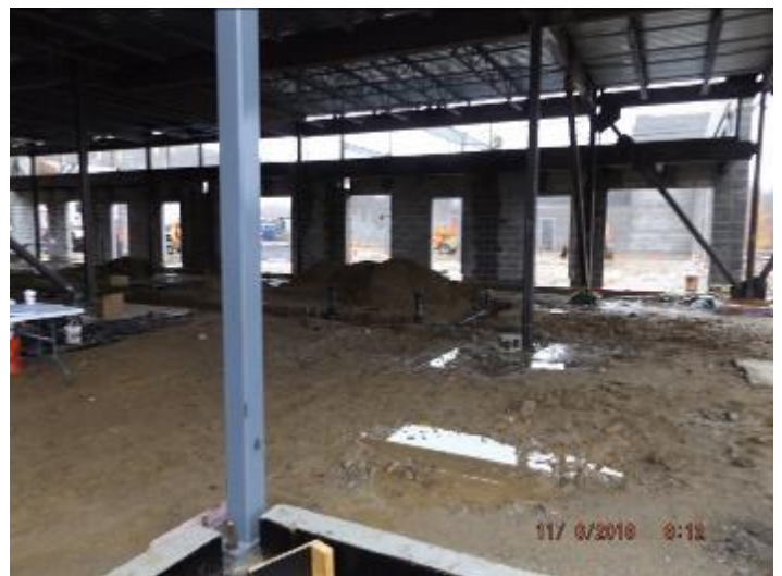
Photo depicts completion of CMU at apparatus bay, and installation of under slab plumbing
