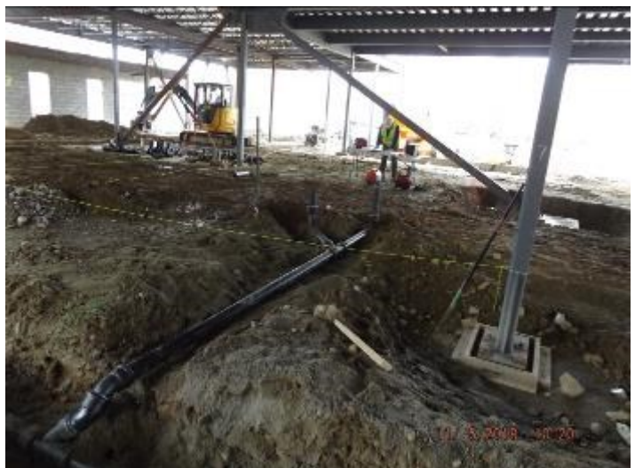
Photo depicts the under slab plumbing installation.
