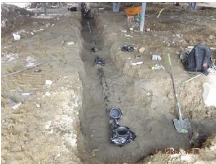
Photo depicts the under slab plumbing installation.
