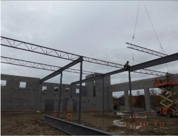
Photo depicts the installation of steel for the apparatus bay roof.
