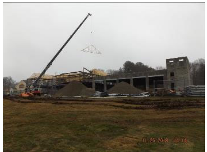
Photo depicts the overall building progress.
