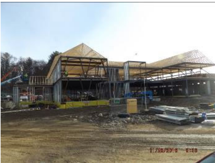
Photo depicts the progress of the roof trusses.
