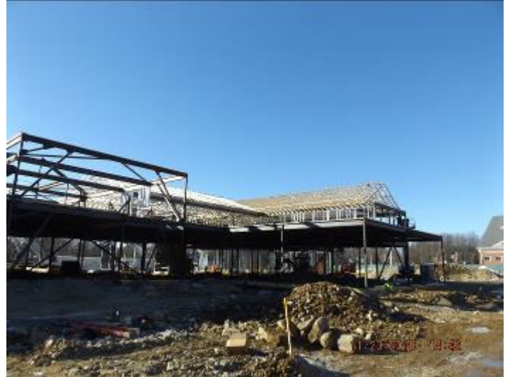
Photo depicts the completion of steel, and installation of roof trusses.
