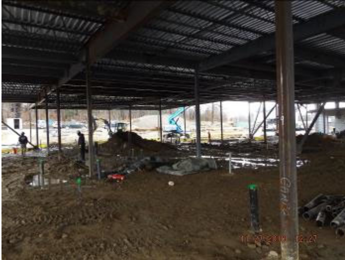
Photo depicts the installation of underground plumbing on police side.
