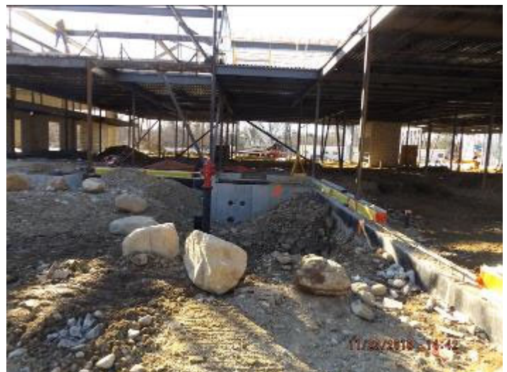
Photo depicts the completed additional hydrant.
