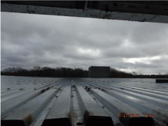
Photo depicts the completed metal deck for the apparatus bay roof.
