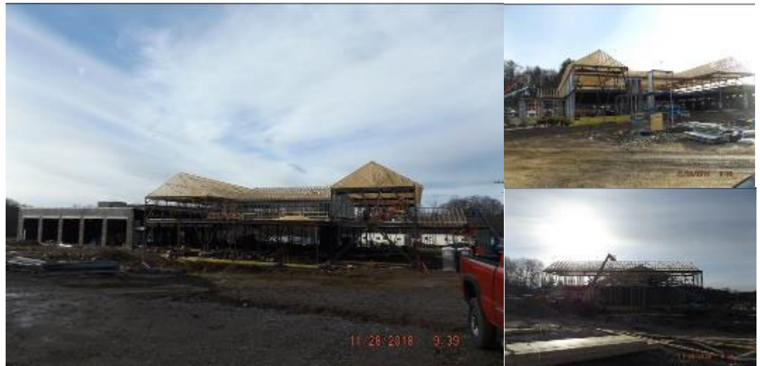
Pictures: Overall building progress
