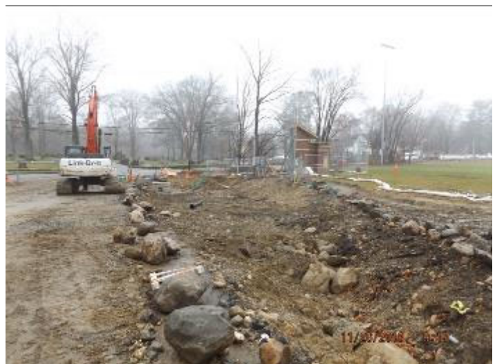
Photo depicts the installation of drainage at future driveway entrance.
