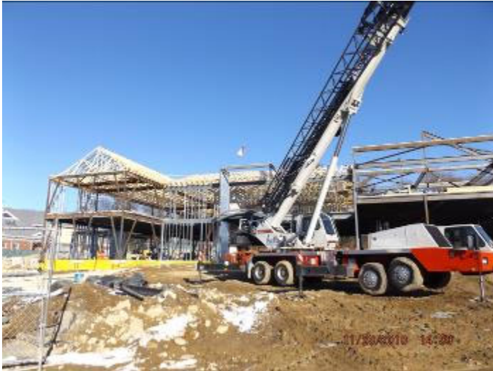
Photo depicts the installation of roof trusses.
