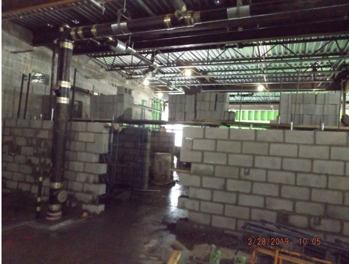
Photo depicts the progress of first floor rough plumbing, electrical, HVAC and CMU walls at the detention area.
