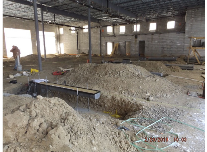
Photo depicts the progress of trench drains in the apparatus bay.
