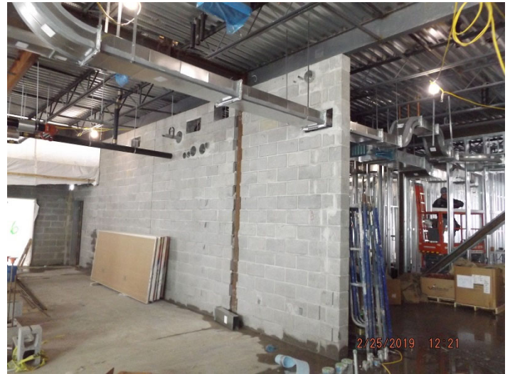
Photo depicts the progress of first floor plumbing, electrical, HVAC and CMU walls at the apparatus bay.
