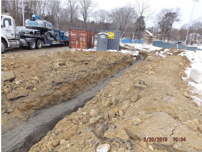
Photo depicts the completion of utility ductbank.
