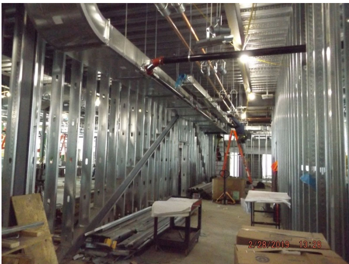
Photo depicts the first floor framing, rough plumbing, electrical and HVAC.
