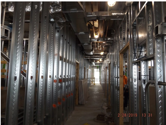
Photo depicts the progress of second floor framing, rough plumbing, electrical and HVAC on Fire side.
