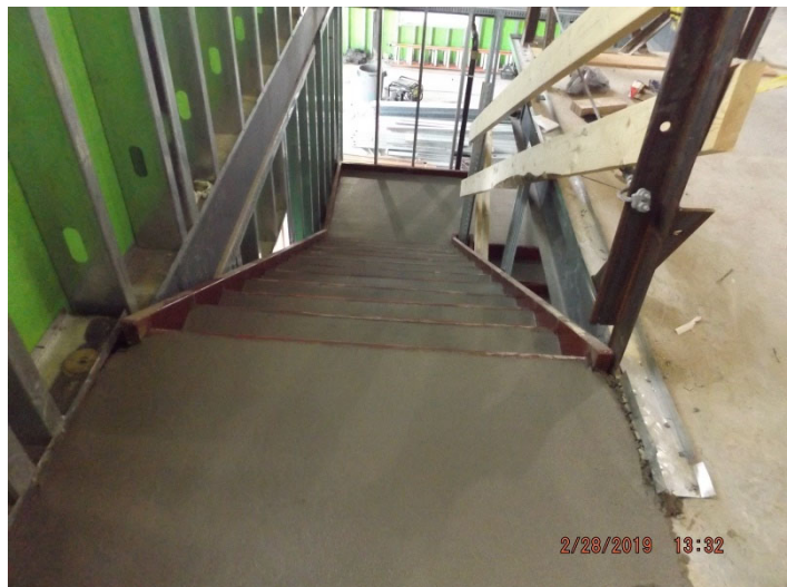
Photo depicts installation of stair #1, complete with concrete.
