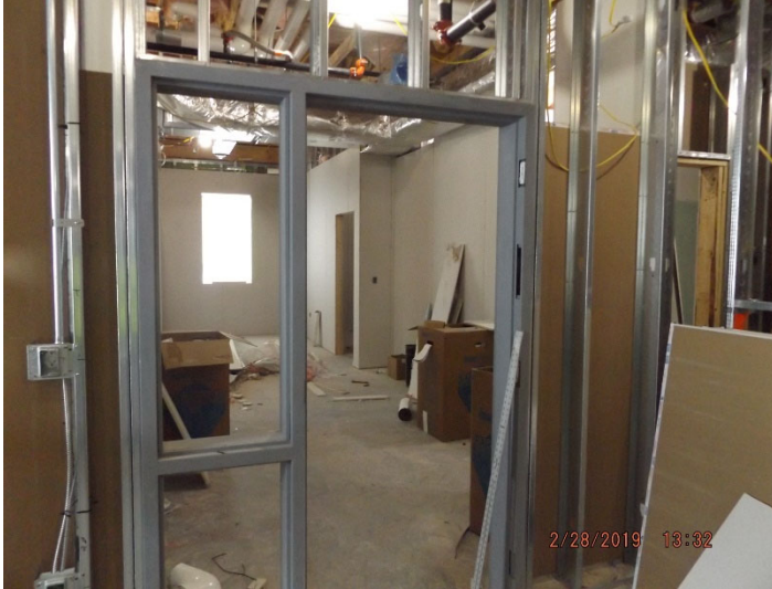
Photo depicts the progress of the second floor framing, drywall, and rough electrical and HVAC on police side.
