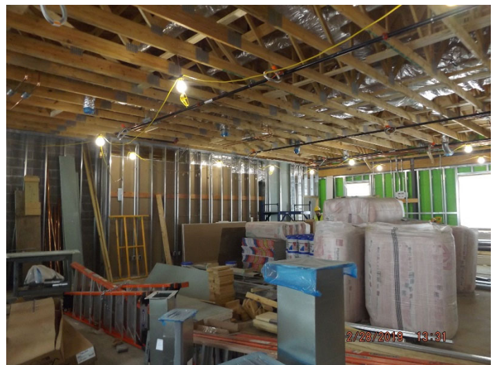
Photo depicts the progress of the second floor framing, electrical, HVAC, and fire suppression in training room.
