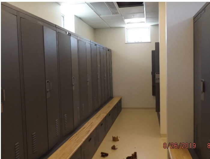
Photo depicts the progress of the police men's locker room.
