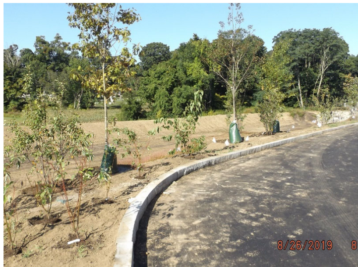
Photo depicts the progress of the landscaping.
