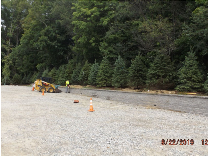
Photo depicts the progress of the landscaping.
