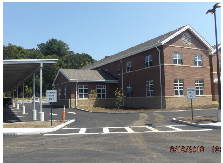
Photo depicts exterior progress at the east side of the building, and the carport.
