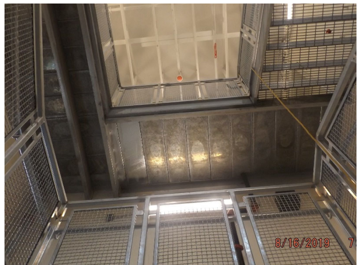
Photo depicts the progress of the training tower stairs and railings.
