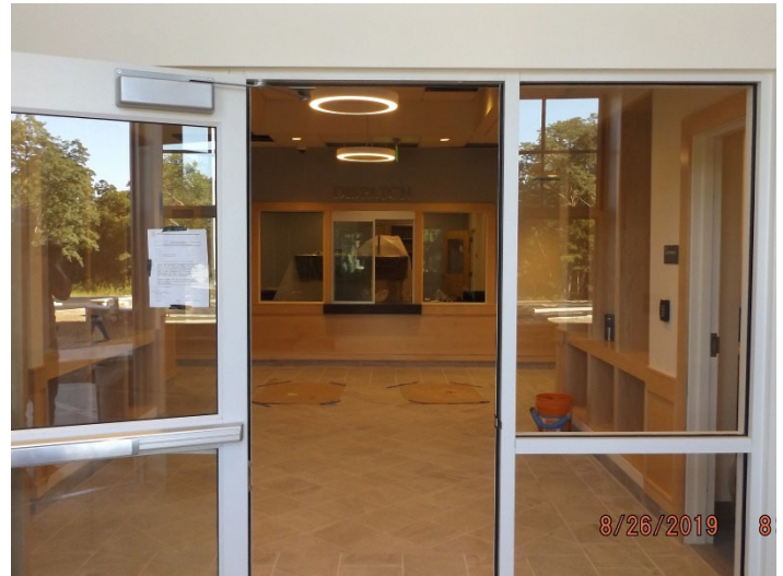
Photo depicts the progress of the main entrance.
