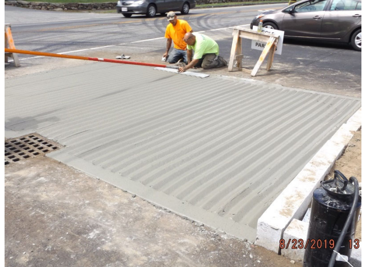
Photo depicts the progress of the rumble strip.
