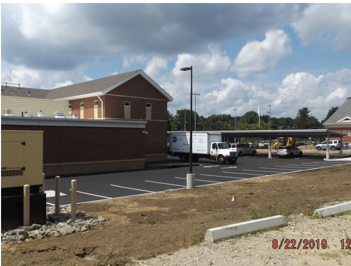
Photo depicts the progress of the exterior of the rear (police side) of building.
