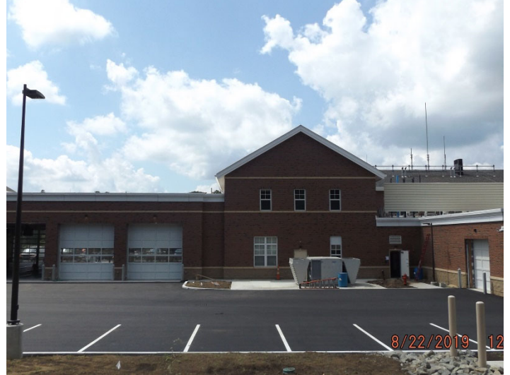
Photo depicts the exterior progress at the rear of the building.
