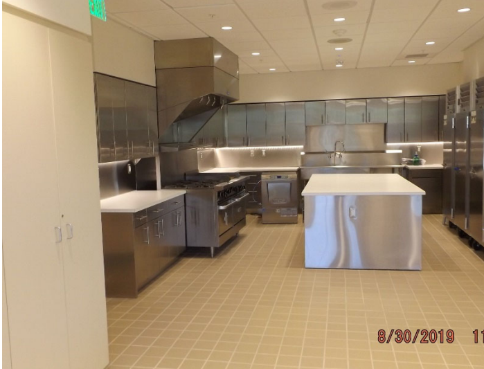
Photo depicts the progress of the Fire fighter's kitchen.
